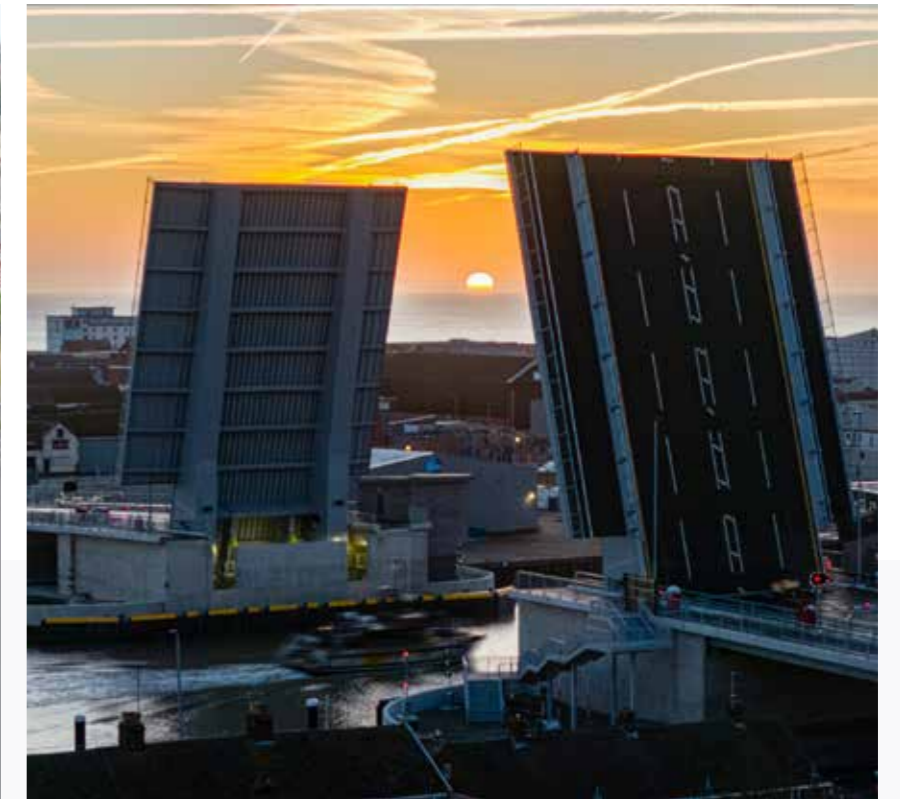
Herring Bridge, Great Yarmouth
