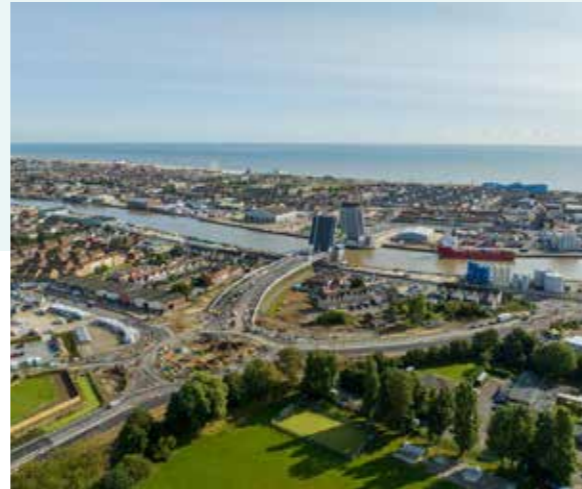
Herring Bridge, Great Yarmouth
